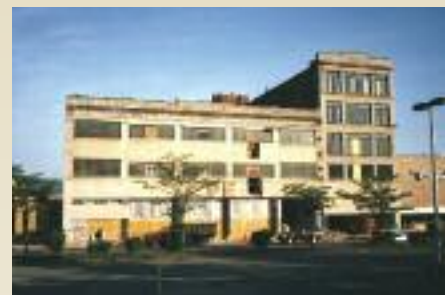
The Discovery Center before rehabbing.
