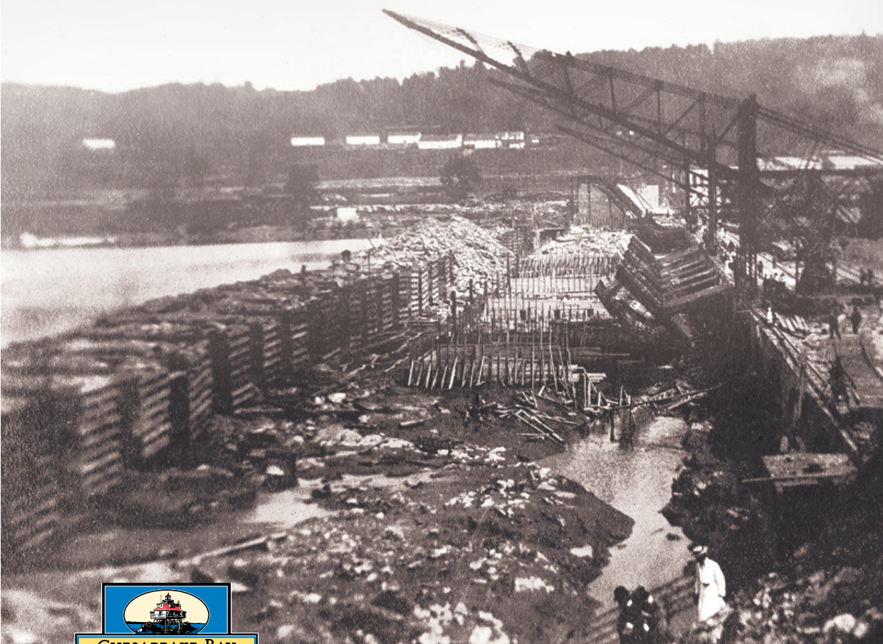
Photo of an early phase of the Holtwood Dam construction project, circa 1906. Note the presence on the left of the "coffer dam" to direct river water away from the construction area.
